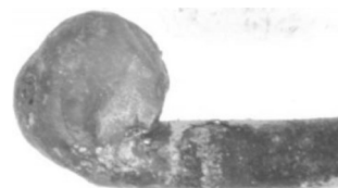
图7 主回路连接线位于弹簧侧断口 Fig. 7 The main circuit connection line located at the spring side fracture
