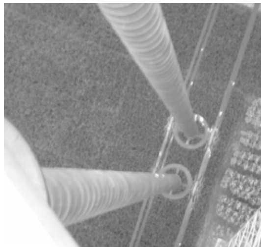
图10 极 I 直流线路故障点导线和绝缘子 Fig. 10 Conductor and insulator at the fault point of pole I DC line
