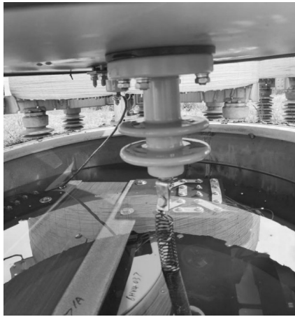
图 5 下节电容单元结构示意图 Fig. 5 Structural schematic diagram of capacitor unit in the lower section
